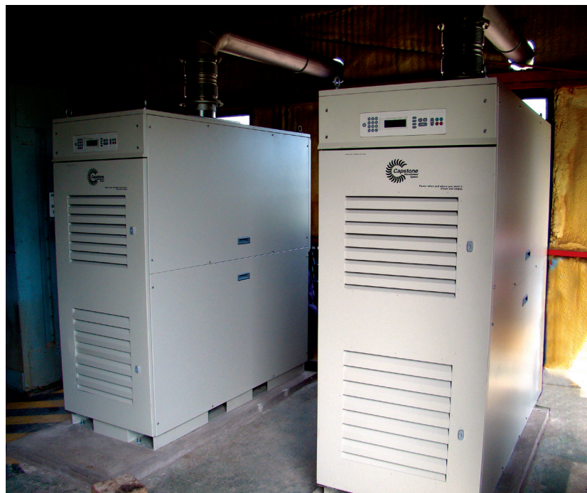
Thirty-five Capstone C65 natural gas-fueled microturbines power compressors at this Bolivian pumping station.
